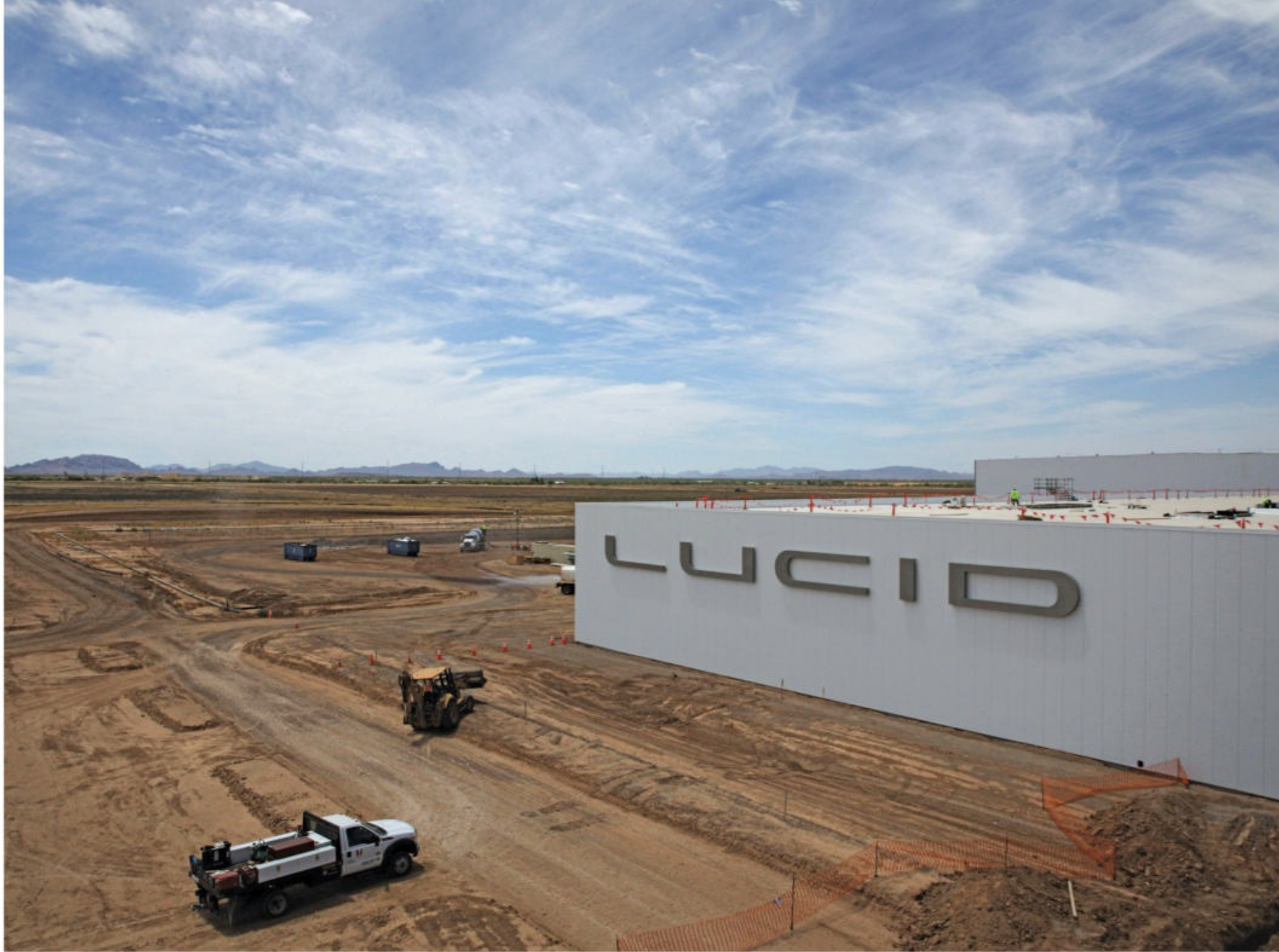
▲ Construction at Lucid's Arizona factory in May 2020
